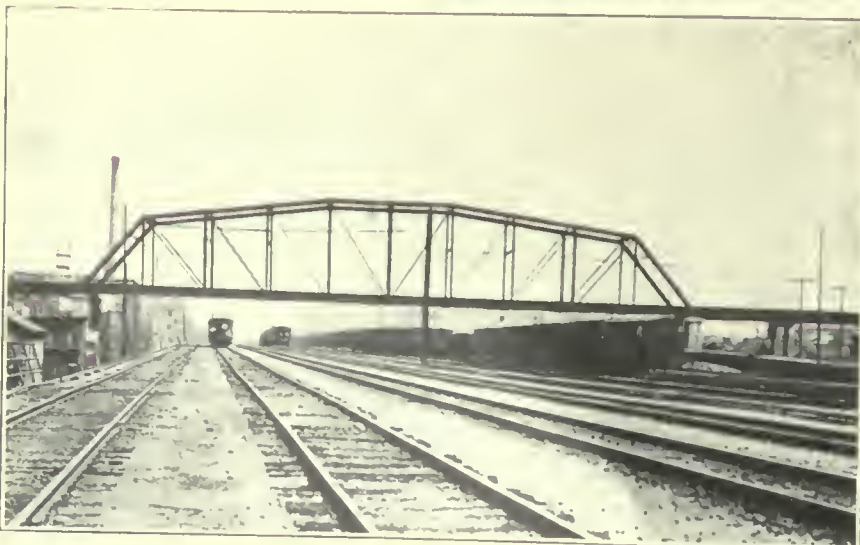
FIG. 269. BRIDGES. Through truss bridge of the Metropolitan Elevated Railway, separating crossing with the Chicago & North Western Railway, the Chicago, Milwaukee & St. Paul Railway and the Pittsburgh, Cincinnati, Chicago & St. Louis Railway.
